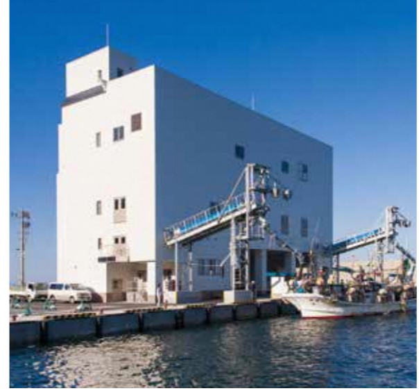
Ice manufacturing plant
